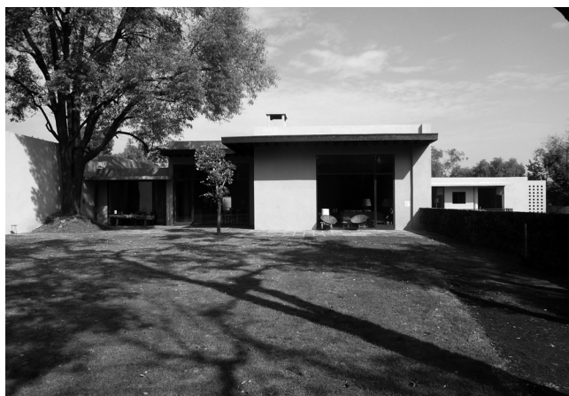
11 Luis Barragán, Casa Pietro Lopez , Pedregal, Mexico, 1950. Restoration by Jorge Covarrubias and Benjamín González Henze, 2014. Facade to the garden. © Louise Noelle, 2014.
