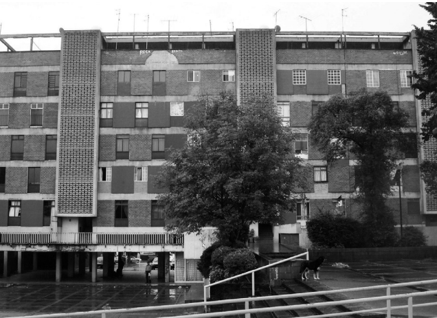
05 Mario Pani, Luis Ramos & Salvador Ortega, Santa Fe Social Services and Housing Unit, Mexico City, 1957. Civic and Social Centre, staircase and 6-floor apartment block. © Juan Pablo Rodríguez Méndez, 2010.
