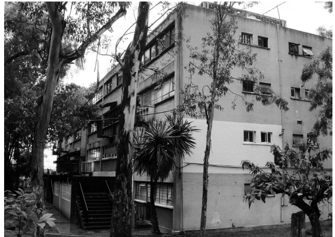
06 Mario Pani, Luis Ramos & Salvador Ortega, Santa Fe Social Services and Housing Unit, Mexico City, 1957. 4-floor apartment block. © Juan Pablo Rodríguez Méndez, 2010.
