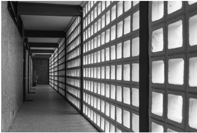
05 Santiago Artal, Santa María Micaela Housing . Cooperative, Valencia, Spain, 1958-1961. Circulation galleries or raised streets. © Ximo Michavila, 2007.
