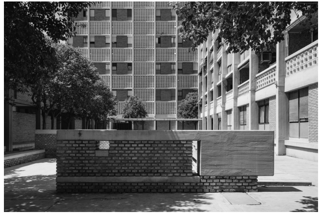
06 Santiago Artal, Santa María Micaela Housing . Cooperative, Valencia, Spain, 1958-1961. Presence of shuttering in circulations and terraces. © Ximo Michavila, 2007.
