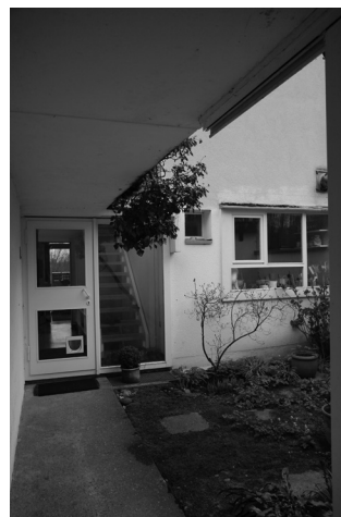
05 Courtyard of the broad type of houses. It is private, but orientated to the pathway, the public space. Beyond the outside door (many inhabitants normally leave it open) the view opens onto the courtyard and to the northern façade. A covered path leads to the entrance. Note the differentiated manners of mounting the windows (from outside, flush mounted, from inside). © Bernhard Furrer, 2012.
