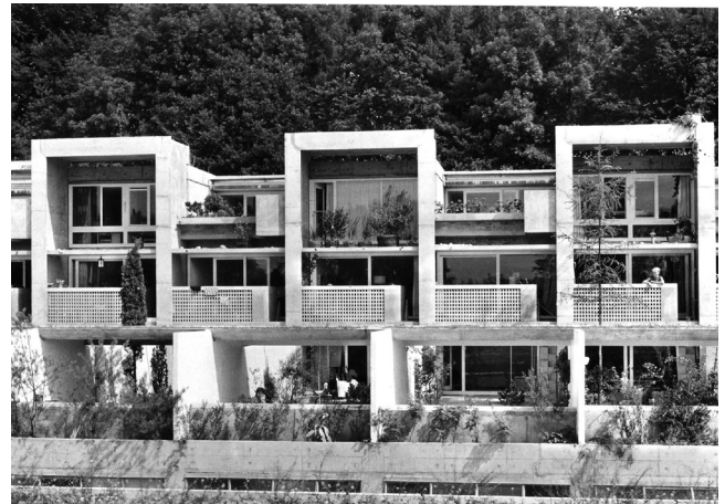
07 Upper western row. The photo taken shortly after completion shows the fresh shiny impression the Estate makes, due to a clear design and to the bright colors (plastered walls, site concrete, concrete elements, windows). The change between houses with and without solarium creates a big variety. © Archive Atelier 5 . Photo by Albert Winkler, 1960s.
