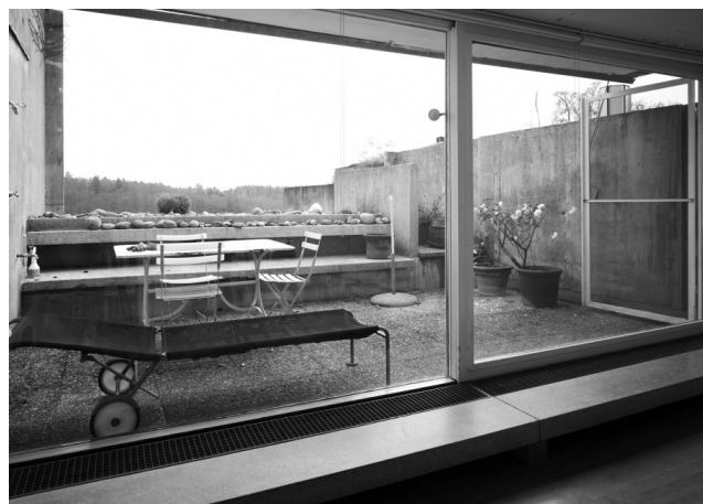
10 Solarium of the broader type of houses. The room behind the solarium opens wide to the outside with a concrete step that hides the convection heater and sliding windows with very slim frames. Towards the south a trough with plants forms a limit to the solarium, a sort of recess permits an overview of the Estate and the landscape. In accordance with the guidelines, covering of the solarium is not allowed anymore. © Archive Atelier 5 . Photo by Nikolaus Schletterer, 1960s.
