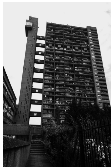
10 Erno Goldfinger, Trellick Tower, Notting Hill, London, 1966-1972. View from Elkstone Road. © Aranzazu Melon, 2014.
