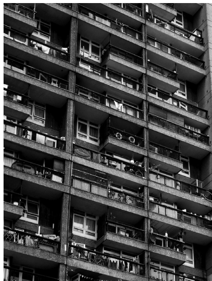
09 Erno Goldfinger, Trellick Tower, Notting Hill, London, 1966-1972. Balconies detail. © Aranzazu Melon, 2014.
