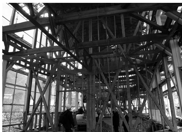
03 Restoration work in progress. © Yoshiaki Hanada, 2009.
