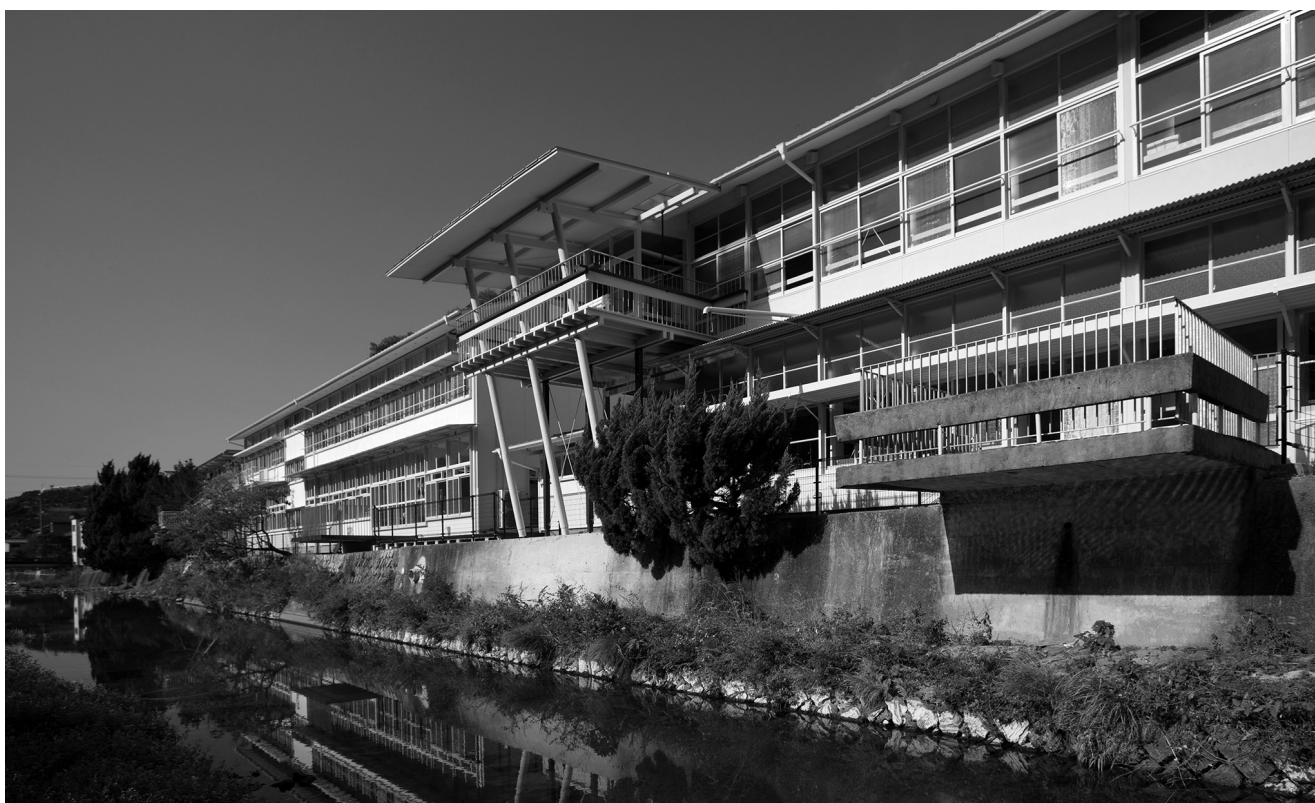
01 General view from south. © Toru Kitamura, 2009.
