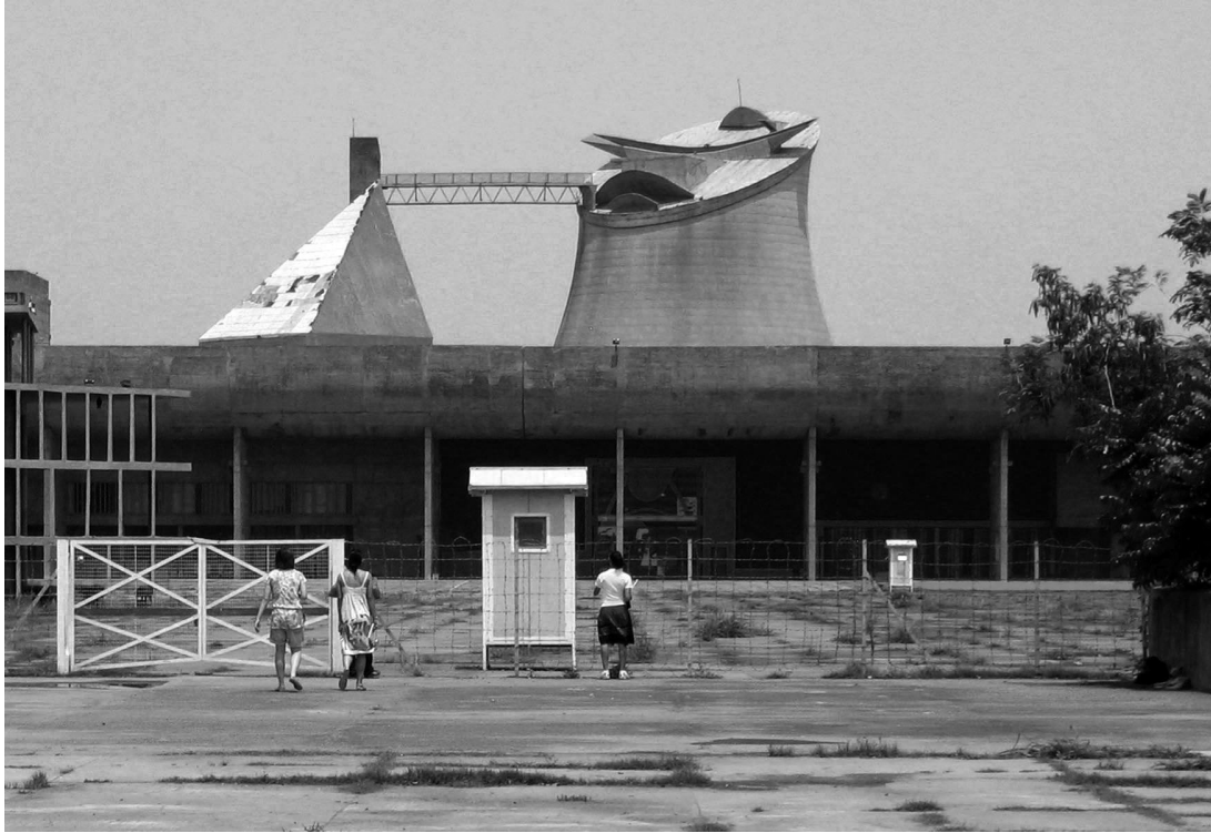
01 Le Corbusier, Assembly Building, Chandigarh, India, 1953-1963. This view from the Esplanade shows the vista interrupted by security fences and guard posts. © 2010 Artists Rights Society (ARS), New York/ADAGP, Paris/FLC, Vinayak Bharne, 2010.
