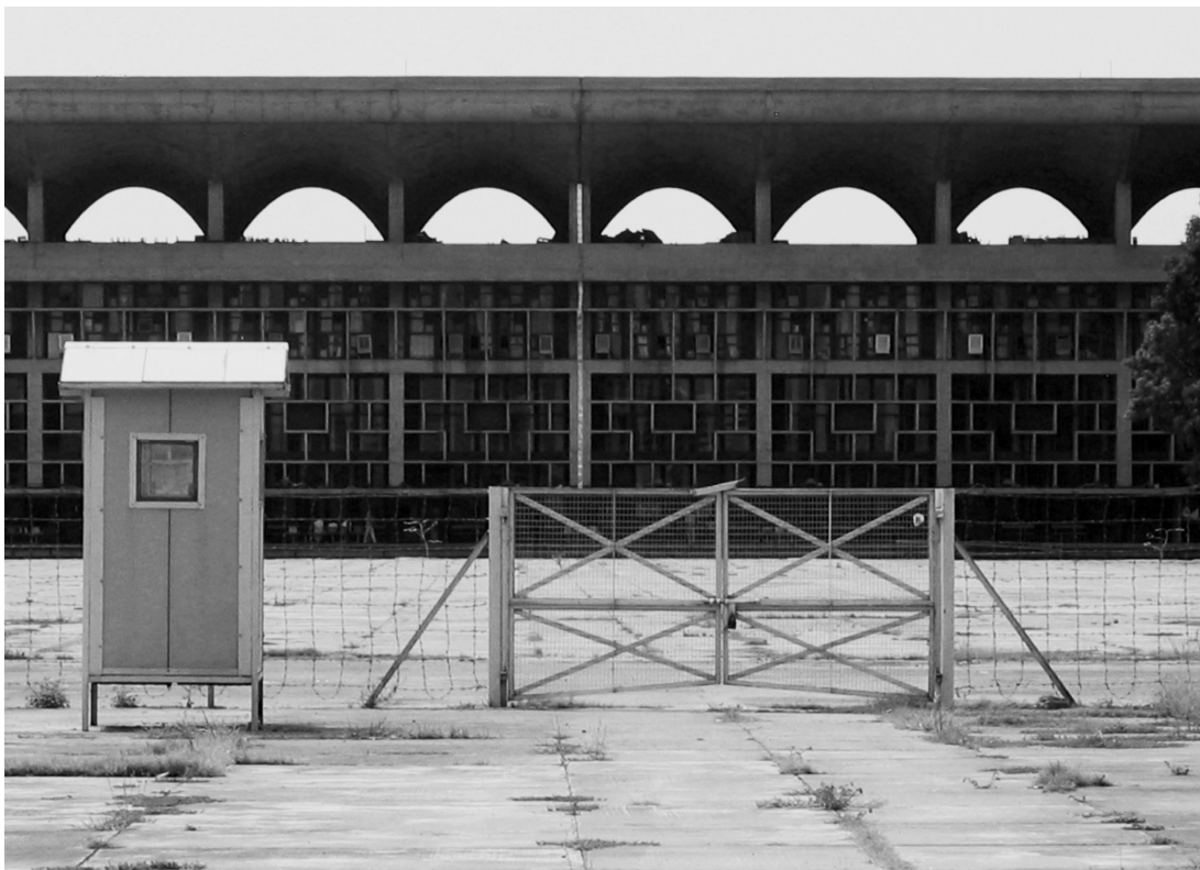
02 Le Corbusier, High Court Building, Chandigarh, India, 1951-1957. This view from the Esplanade shows the vista interrupted by security fences and guard posts. © 2010 Artists Rights Society (ARS), New York/ADAGP, Paris/FLC, Vinayak Bharne, 2010.
