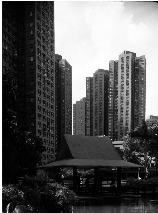
10 Siu Hong Court, Tuen Mun New Town, Hong Kong, 1981-1985: one of the HKHA's largest Home Ownership Scheme developments. The standard HOS towers were designed by architects of the Housing Department Construction Branch, and the project was opened in 1985 by Chief Secretary Sir Philip Haddon-Cave. © Miles Glendinning, 2012.
