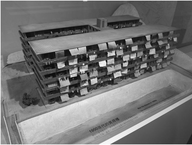
01 “Mark 1” Resettlement block as built 1954 at Shek Kip Mei, Hong Kong: reconstruction model housed in Mei Ho House, the last surviving Mk. 1 block, converted after 2011 to a heritage centre and youth hostel. © Miles Glendinning, 2014.
