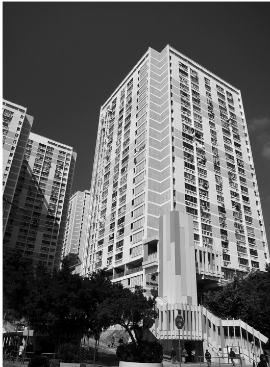
09 Wah Fu Estate, Hong Kong: "twin tower" blocks designed by Donald Liao and his staff in 1965 and built by the "old" HKHA in the late 1960s and early 70s on this dramatic sea-panorama site. This view shows part of the Wah Fu (II) estate, opened between 1970 and 1978. © Miles Glendinning, 2014.
