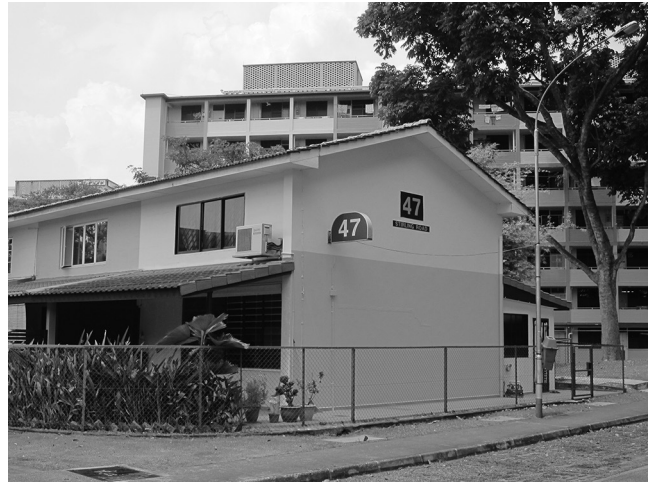
02 Queenstown Neighbourhood 2 (Duchess Estate), late 1950s low-rise blocks designed by the architectural staff of SIT: the flats in the background (blocks 45, 48, 49) were the first completed by the HDB, in 1960. © Miles Glendinning, 2011.
