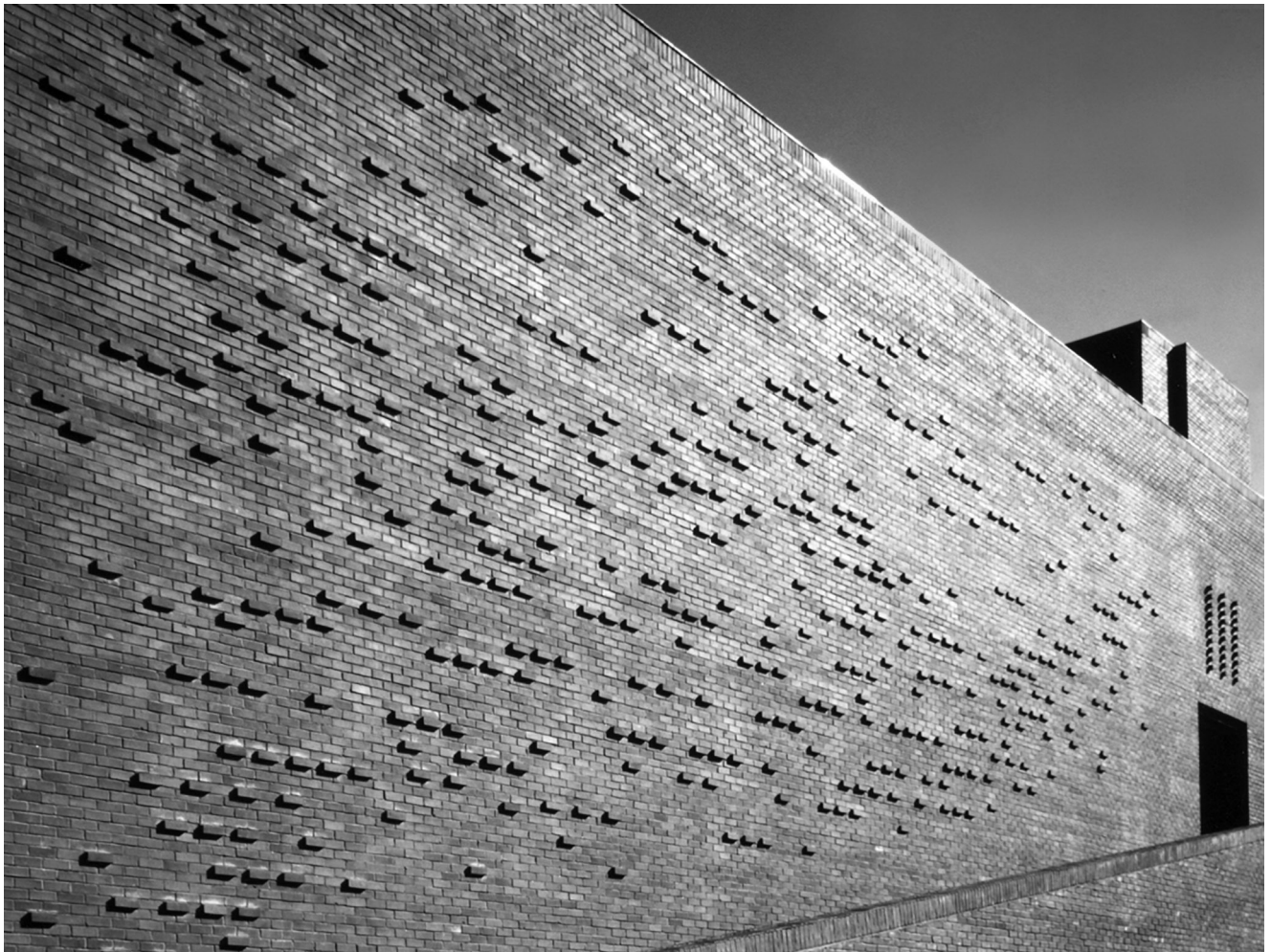
10 Swoo-Geun Kim, Arko Gallery, Daehangno, Seoul, South Korea, 1977-1979. Brick details. © In Space Magazine, Jan. 1980, p. 76
