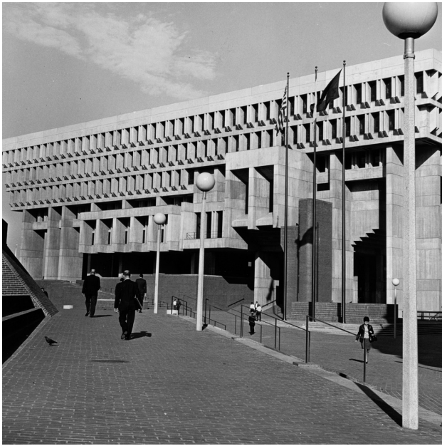
Figure 1. Boston City Hall, vilified on completion as “a giant concrete harmonica” a “pigeon cage,” or an “Aztec gas station.”
