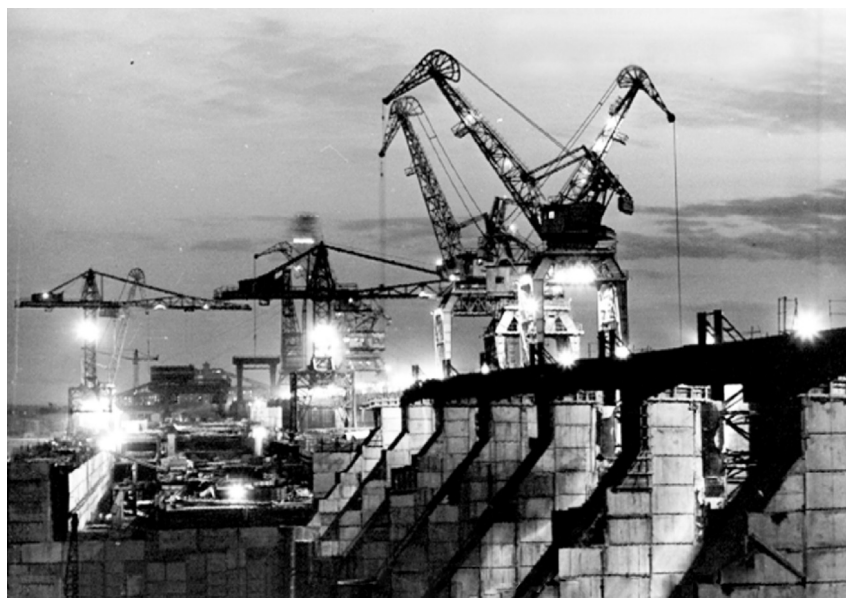
Figure 1. Kremenchug Hydroelectric Power Plant, Svetlovodsk, October 2, 1959.
