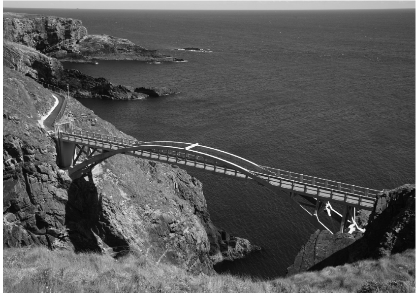
Images of the New Mizen Bridge completed in 2010.
