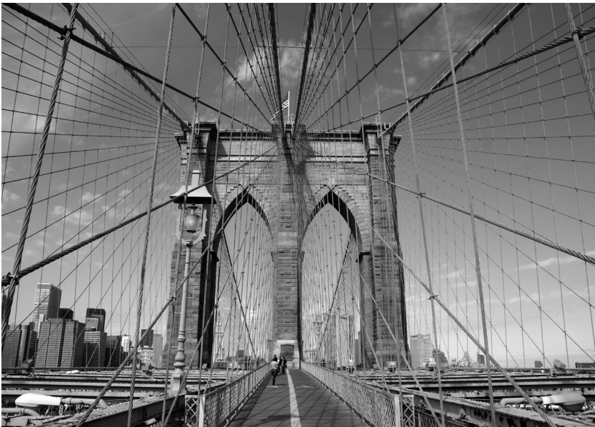
Figure 1. The impressive net generated by the vertical hangers and the diagonal stay cables of the Brooklyn Bridge, New York, by John August Roebling , 1883.
