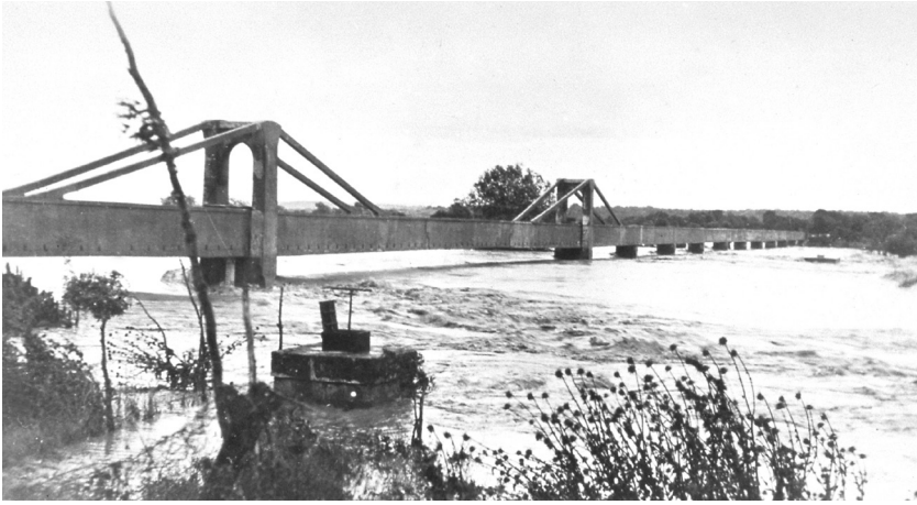
The Tempul Aqueduct during a flash flood.
