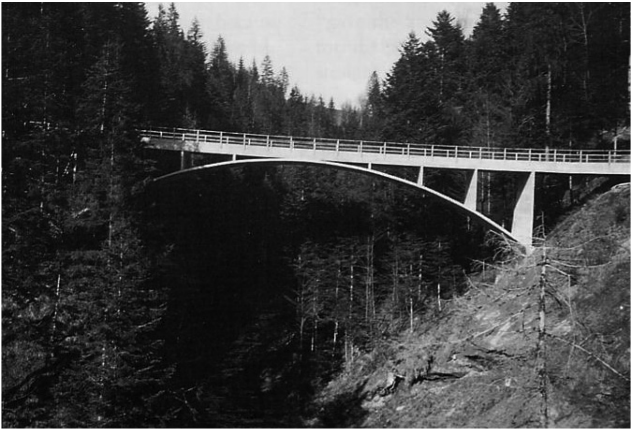
Figure 1. Maillart's reinforced concrete arch Schwandbach Bridge near Berne, built in 1933.
