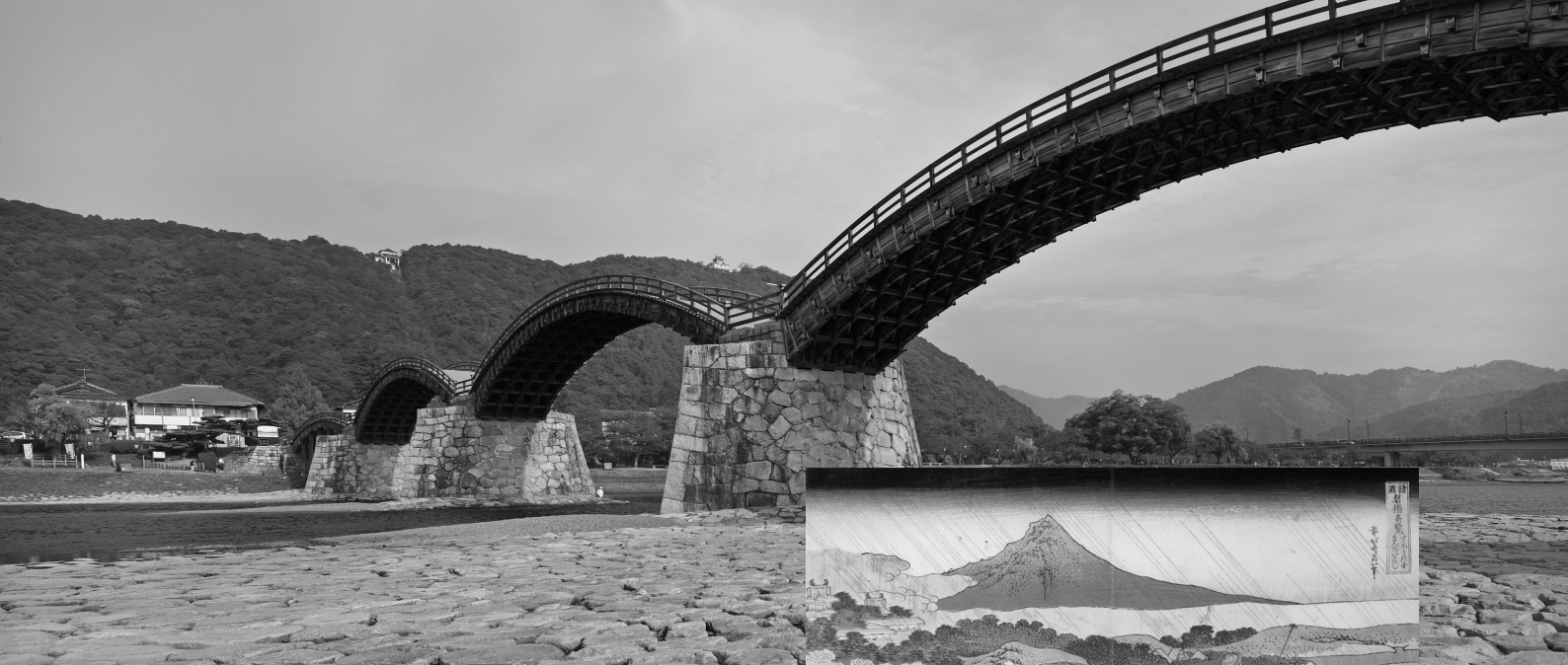
The Kintai Bridge today. Photo by Jens Markus Lindhe.
